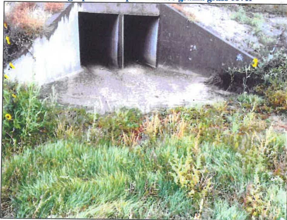
Photograph A-4. Drainage from parcel exits property and continues northeast through Route 66 box culverts
